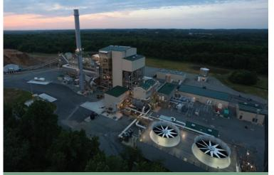
ince November 2013, NOVEC's 49-megawatt biomass plant has been producing environmentally-friendly electricity using waste wood from logging operations as the primary fuel source. This waste wood (the part of the tree that has no commercial value) previously was either left in piles to decompose, which produced methane -a harmful greenhouse gas – or burned on the property where the logging activity occurred. Now that waste wood is used to produce green energy.
