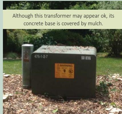
Although this transformer may appear ok, its concrete base is covered by mulch.
